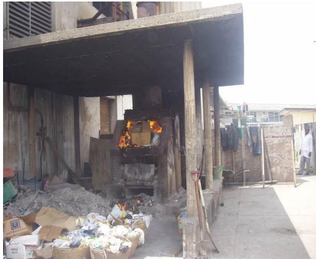
**Picture 12: A locally built incinerator at a healthcare facility, Ibadan, Nigeria**
