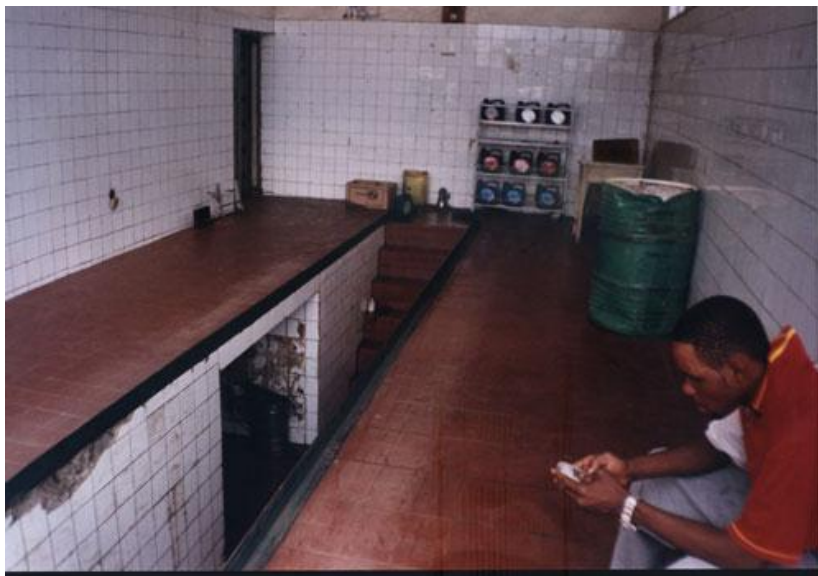
Fig 3.2: A well managed service station bay for oil change
