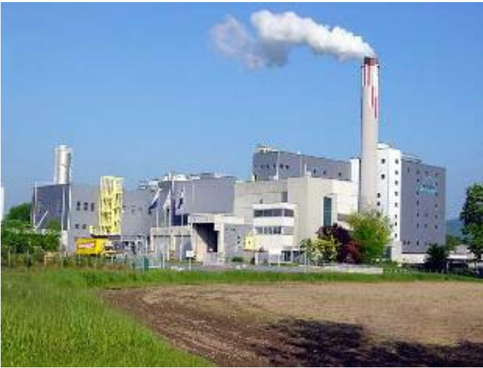
Figure 16. Municipal Solid Waste Incineration Plant
