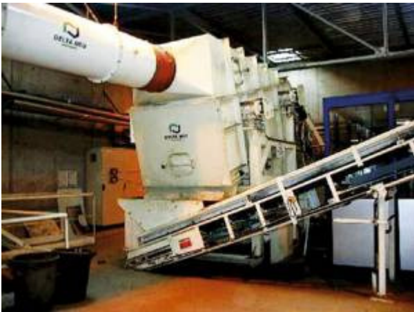
Figure 19. Waste sorting machine designed by TRISELEC.
